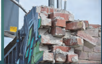
Figure 6: Example of weak mortar from damaged building.
