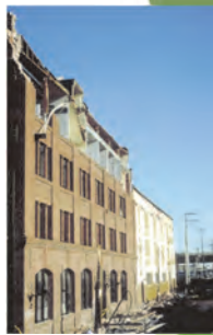
1989 Loma Prieta. 5 People died. Photo Credit: James Blacklock, WGBH-TV, Berkeley
