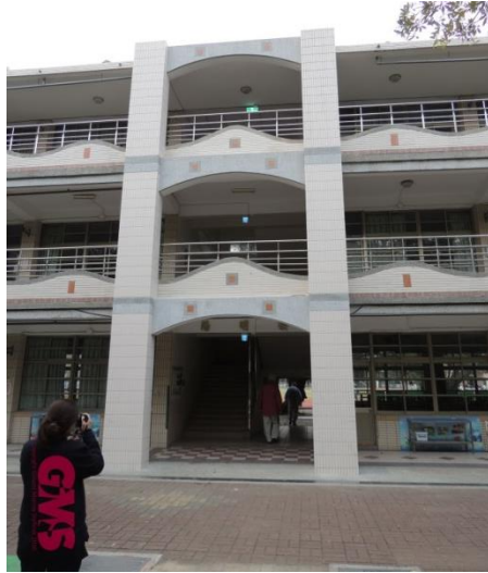
Figure 6: Guiren Middle School Retrofitted with Added Moment Frame (Minor Damage)
