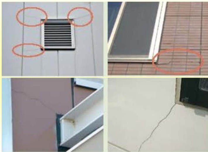
Example of tiles to be loosed
