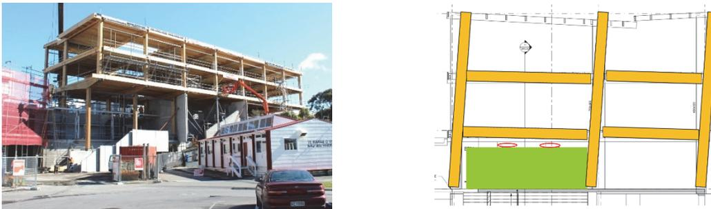
Figure 6. External view during construction and diagram of rocking frame and damper arrangement.
