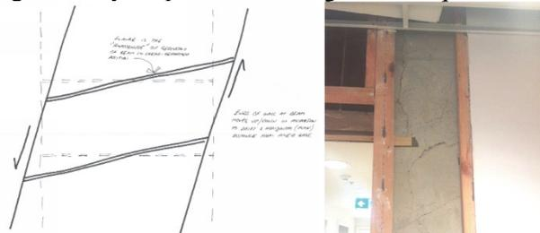
Figure 11. Diagram of elongation demands and cracking at the cast-in coupling beam ends at The Customhouse.
