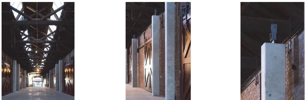
Figure 1. Internal space of Shed 13 showing new frame and detail of ductile link to roof trusses.
