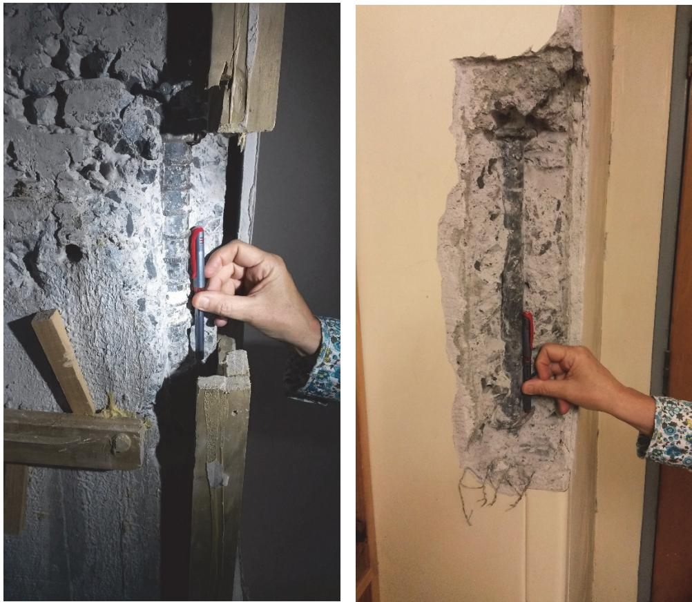
*Figure 5. Deformed bar used in half of the building, and round bar being used in the other half.*
