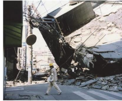
Photo 3. Collapse of building on a road.
