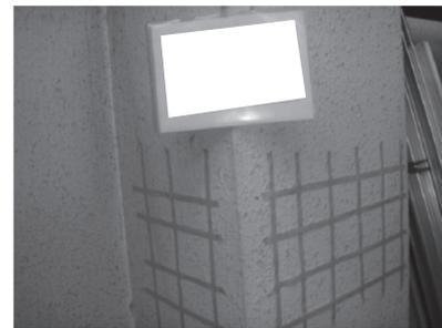
Photo 5. Marking of re-bar arrangement.
