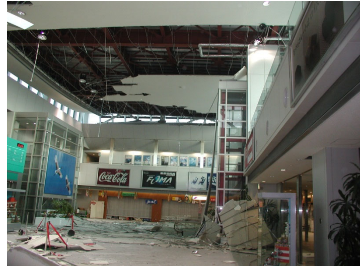
Falling down of suspended ceiling in the airport terminal building (2003 Off Tokachi Earthquake)
