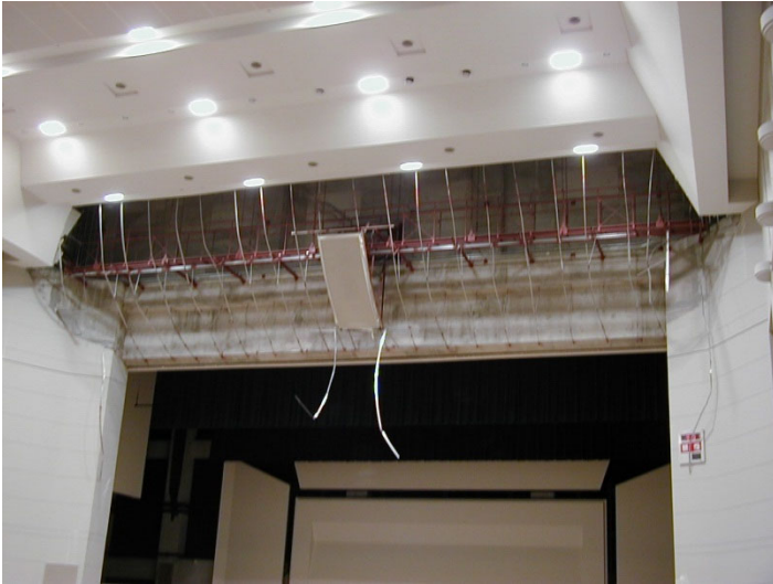
Falling down of suspended ceiling in the gymnasium (2001 Geiyo Earthquake)
