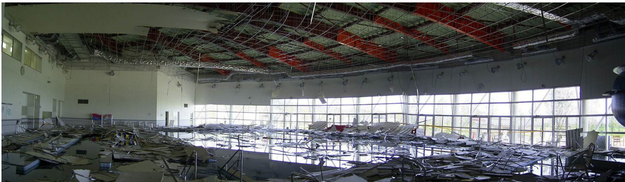
Falling down of suspended ceiling in the indoor swimming pool (2005 Off Miyagi Prefecture Earthquake)
