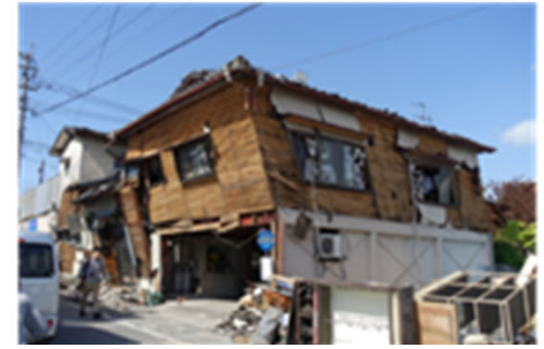
Second floor hugely tilted in a S+W house
