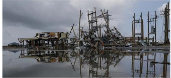
Electric and power
