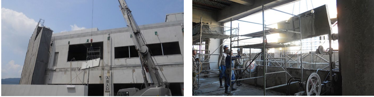
Figure 7. Demolition Process Using Disk Sawing Method.
