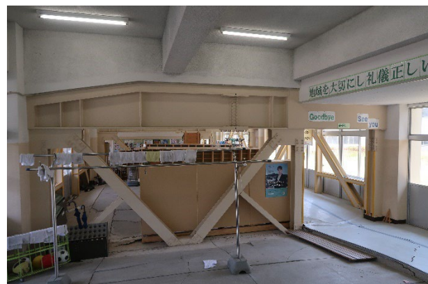
Figure 5. Seismic retrofit of building C-1
