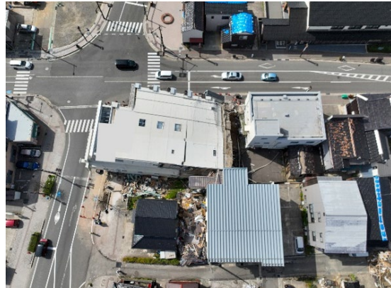
Figure 13. The building AA (West side)
