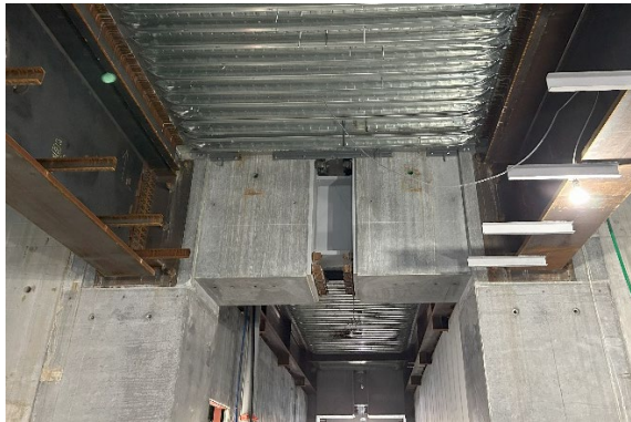
(a) Damping beams between core walls
