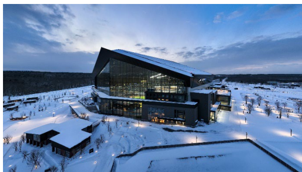
Figure 1. Exterior view in winter
