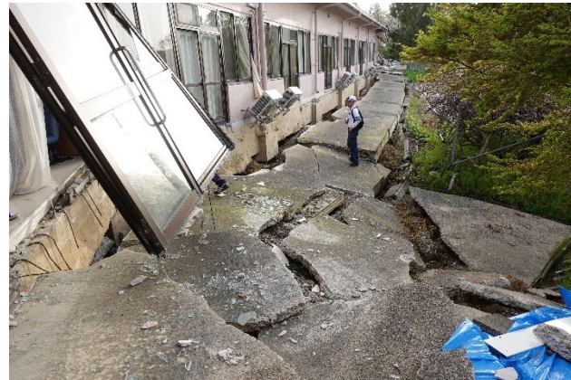
Figure 22. Ground deformation
