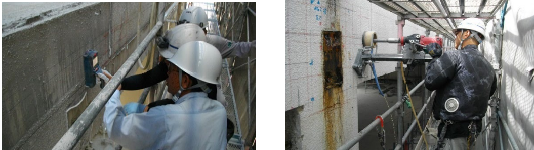
Figure 10. Rebar Location Scanning and Drilling Process During Construction.
