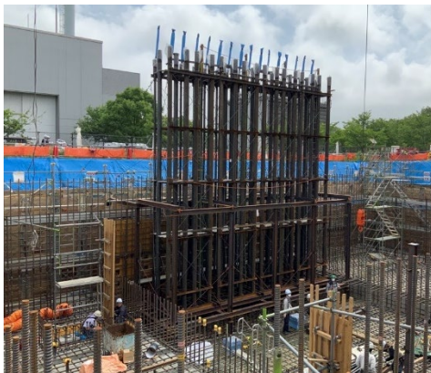
(a) Template framework for sheath tube
