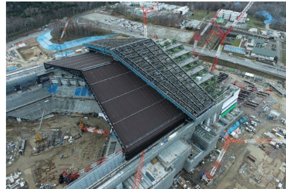
Figure 16. process of jacking up retractable roof from fixed roof
