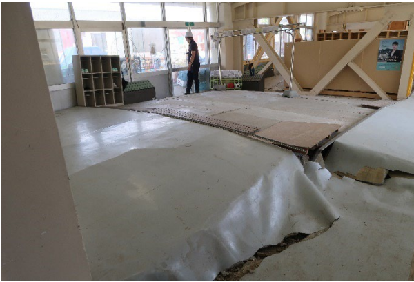
Figure 6. The undulation of the first floor
