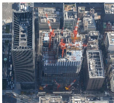
(b) Construction status photo(Nov. 2023)
