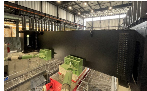
(c) Installed reaction beam on elastomeric bearings
