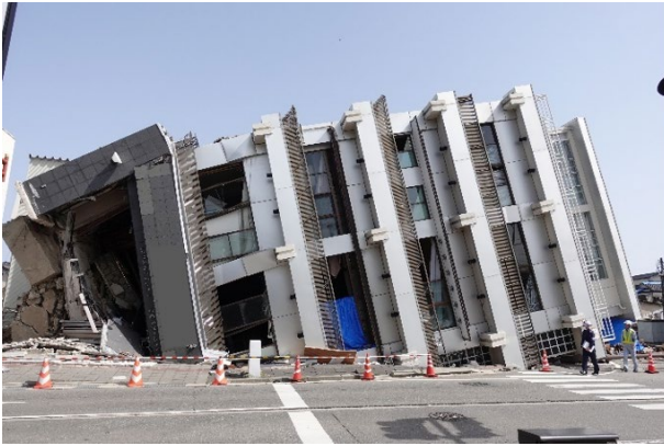
Figure 12. The building AA (South side)
