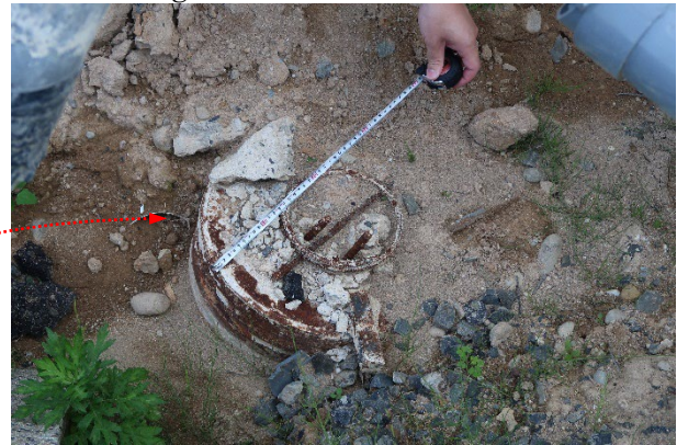
Figure 11. Exposed cross section of pile head
