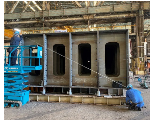
(b) Fabrication of reaction beam
