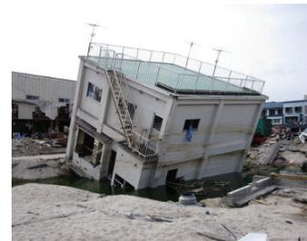
Figure 12. Tilting by scouring
