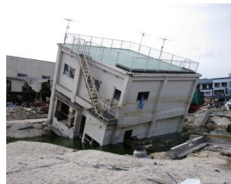
Figure 12. Tilting by scouring
