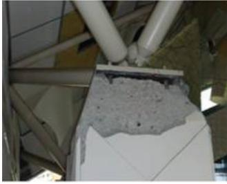
Figure 4. Spalling of concrete
