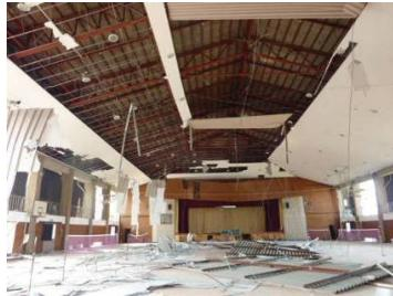
Figure 5. Fallen down of ceiling
