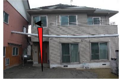
Figure 9. Tilted house by liquefaction
