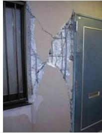
Figure 7. Nonstructural wall failure
