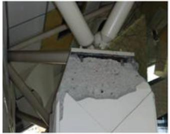
Figure 4. Spalling of concrete
