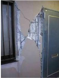
Figure 7. Nonstructural wall failure
