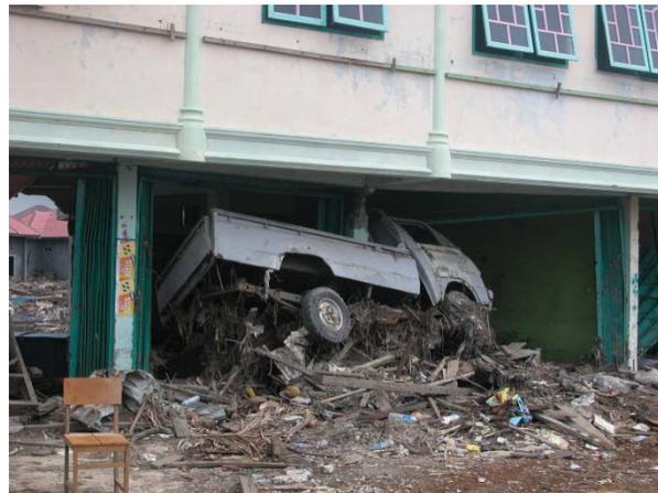
Figure 2-16 Examples of waterborne debris from the 2004 Indian Ocean Tsunami (photos courtesy of M. Saatcioglu, A. Ghojarah and I. Nistor, CAEE, 2005).
