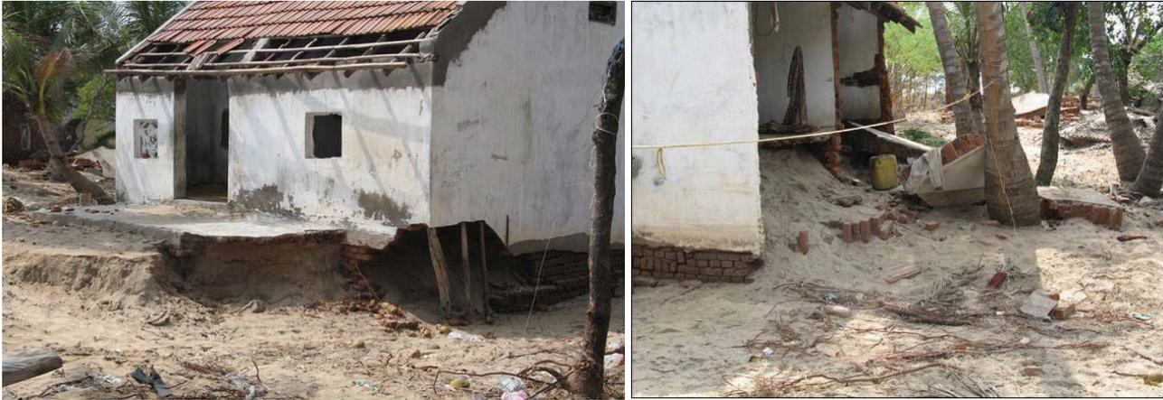
Figure 2-14 Damaged masonry beach house in Devanaanpattinam, India (2004 Indian Ocean Tsunami).
